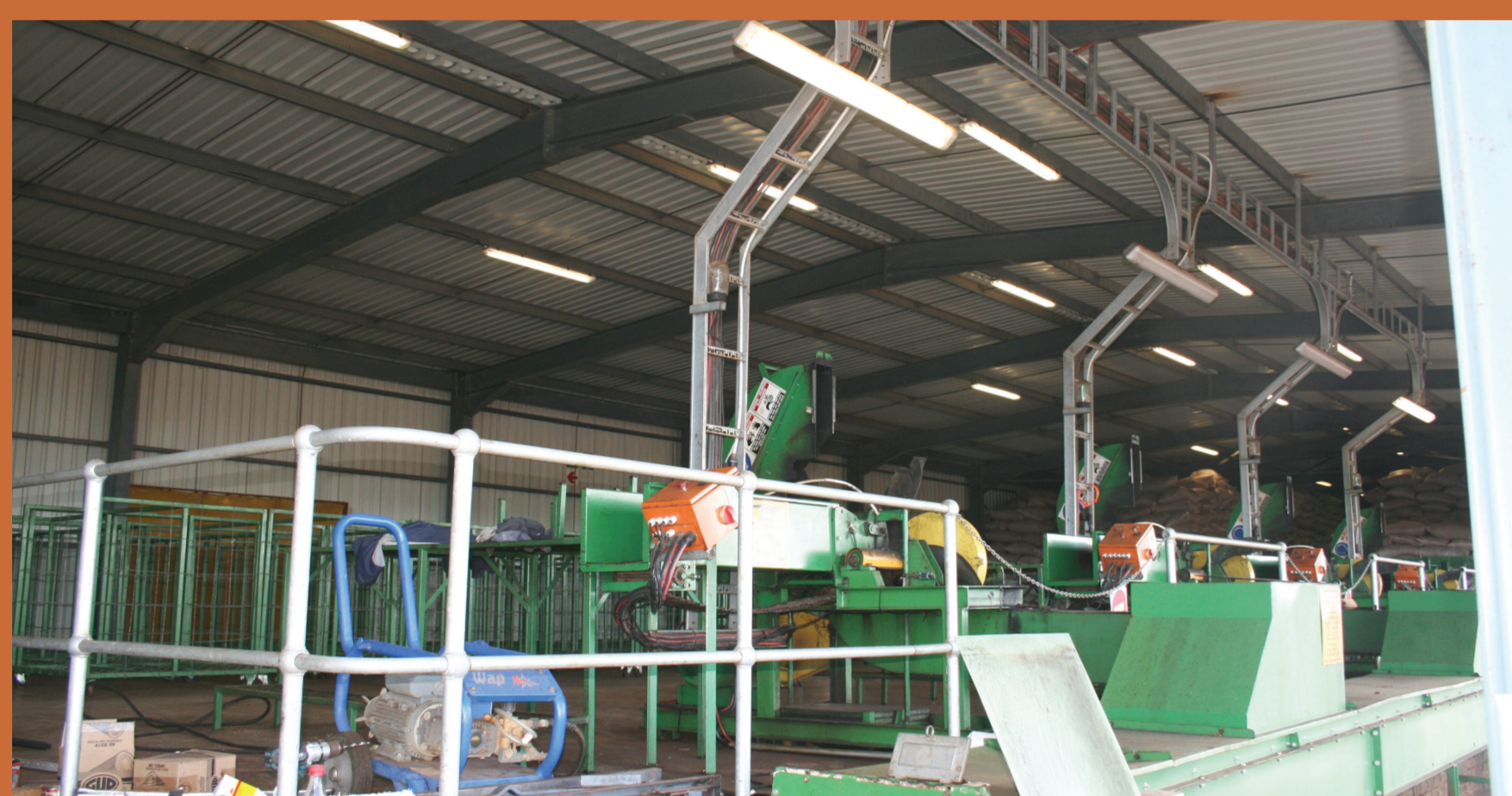
Rooibos tea processing facilities
